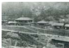
Company's office in the Motoyama District
