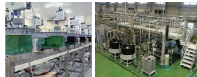
Bench-scale equipment at Hitachi Works Demonstration testing equipment at Tsuruga Plant
