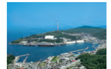
Saganoseki Smelter & Refinery, JX Metals Smelting Co., Ltd.
