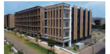
The Material Innovation Center
