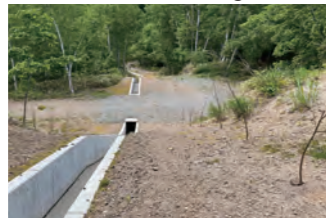
The drainage canal of the Toyoha Mine Ishiyama tailings dam, completed in FY2022
